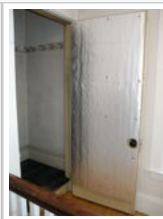
Air leakage at doors leading to unconditioned space and typical solution:
