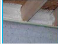
Remove existing fiberglass if present in box sills and replace with either spray foam or rigid foam. If rigid foam is utilized, care should be taken to assure complete air sealing of box sills and top plate(s).
