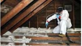
Any attic work must first start with creating a comprehensive air barrier along the attic floor. In many homes, especially older homes with plaster and lathe, the best way to fully seal the attic flat is with a continuous layer of closed cell spray foam.
