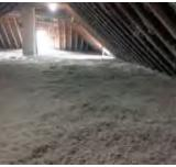
A thick blanket of cellulose can be installed after air sealing to bring your attic to the R50 energy code and beyond. Cellulose is a recycled newspaper product and is treated to be both fire and rodent resistant. The image on the left is your attic and the image on the right is what your attic might look like after an insulation upgrade project.
